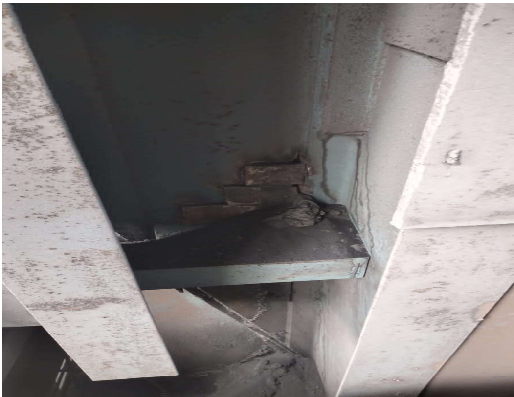
Bunker Hopper coal leakages
