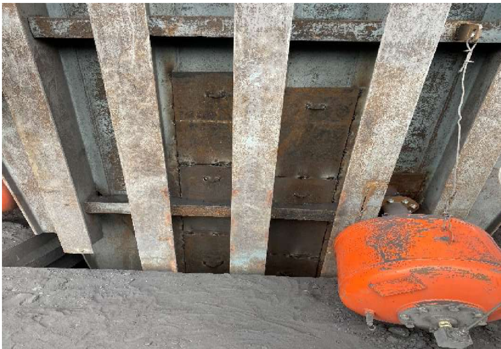
Bunker Hopper damaged
