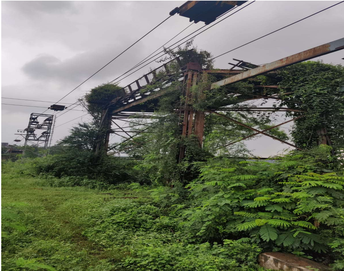
Ropeway rusted steel structure
