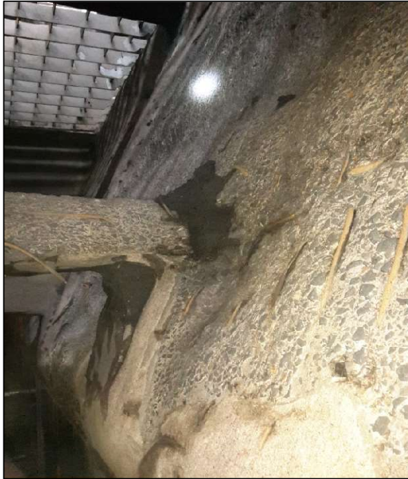
WT RCC Hopper damaged
