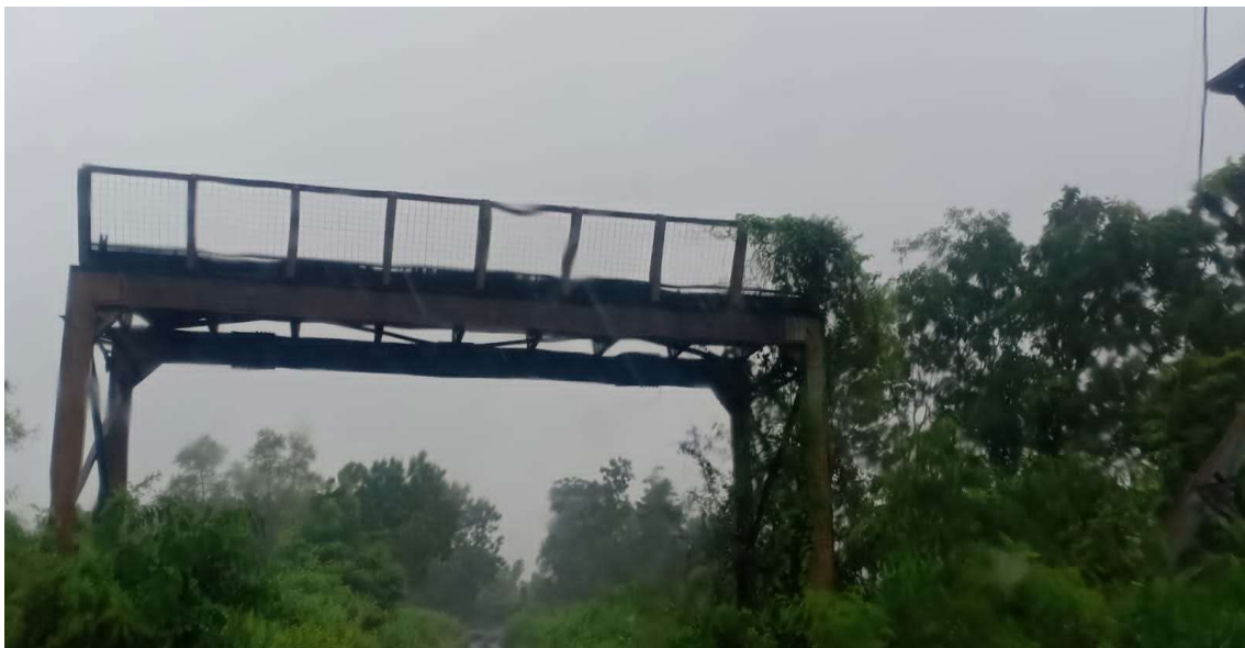
Rusted Ropeway OHE crossing platform
