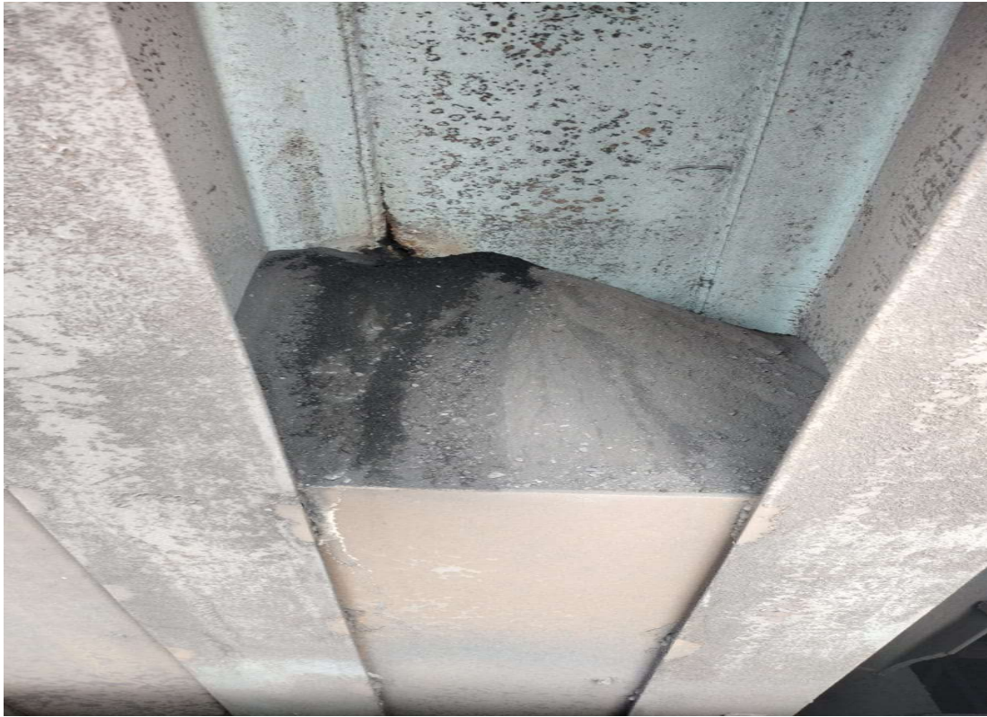
Bunker Hopper coal leakages
