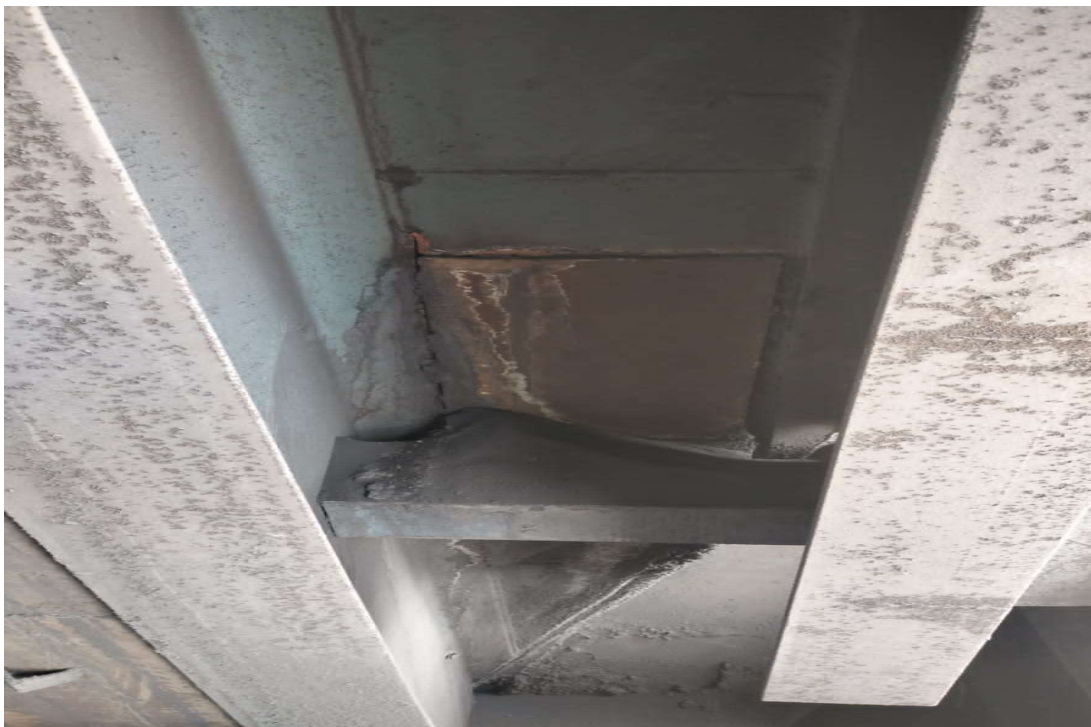
Bunker Hopper damaged
