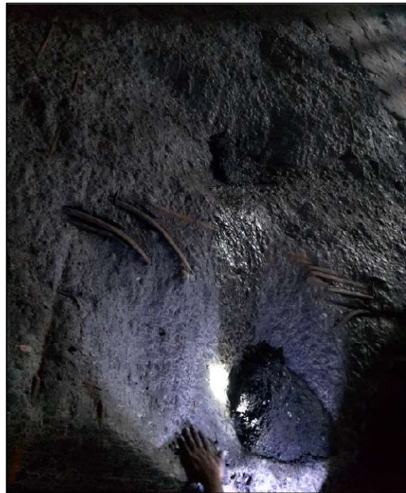
WT RCC Hopper damaged
